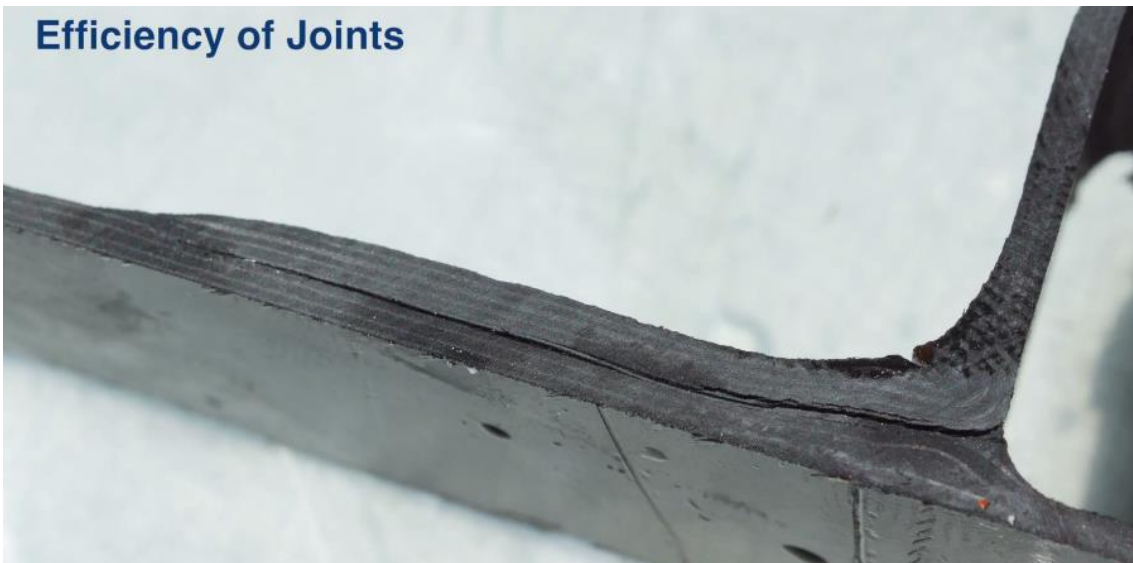
Figure 31 - The joint strength in composites is not very good. So you should design a large part in order to minimize the number of joints.
