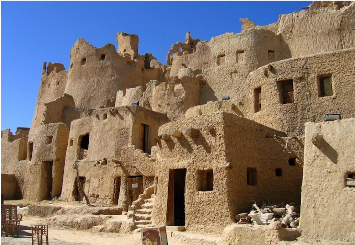
Figure 1 Houses made with mud bricks in Siwa Oasis, Egypt
