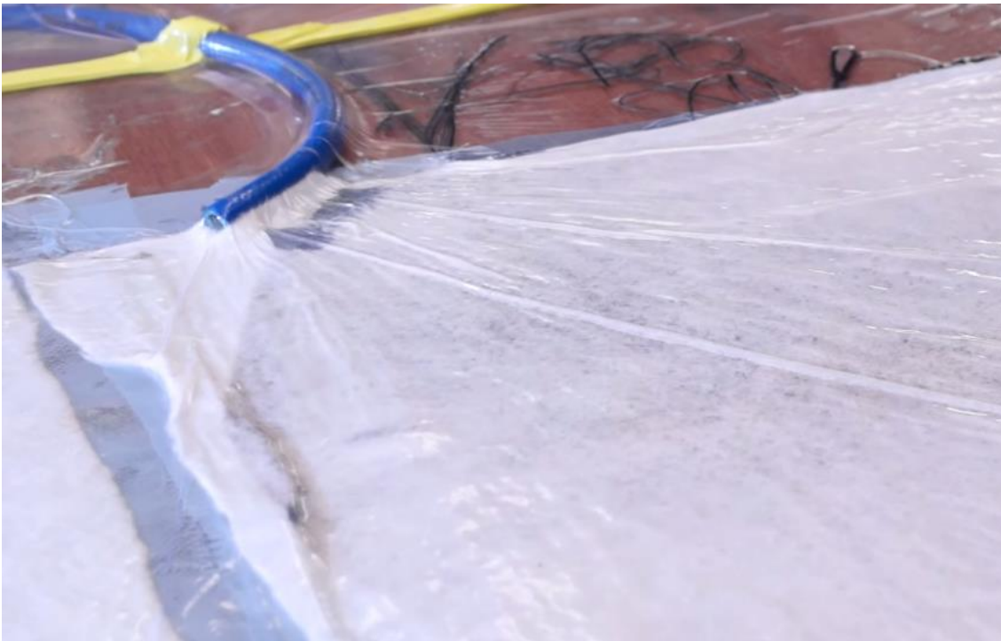
Figure 24 - applying vacuum to get rid of air bubbles and volatiles
