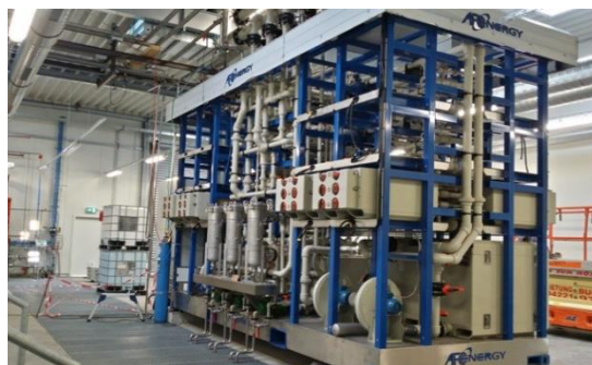
Fig. 44 AFC Energy's "POWER-UP", the world's largest operational AFC system at Air Products' industrial gas plant in Germany (1).
